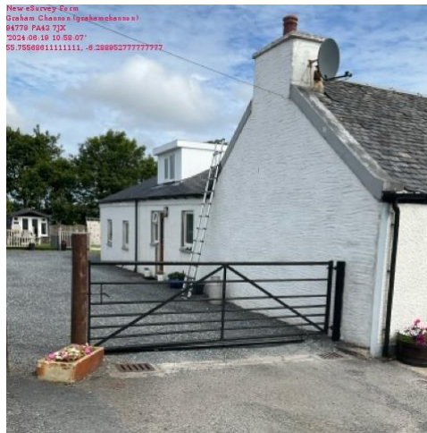
No1 Dairy Cottage – West Facing Gable Elevation
