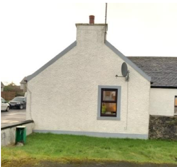
No2 Dairy Cottage - East Facing Gable Elevation
