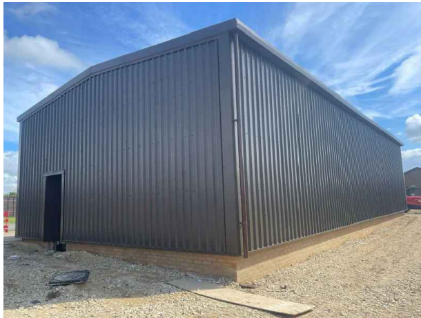
Example of: metal cladding to be non-drip - Colour - Green on 215mm blockwork with steel framed access doors & up and over roller door
