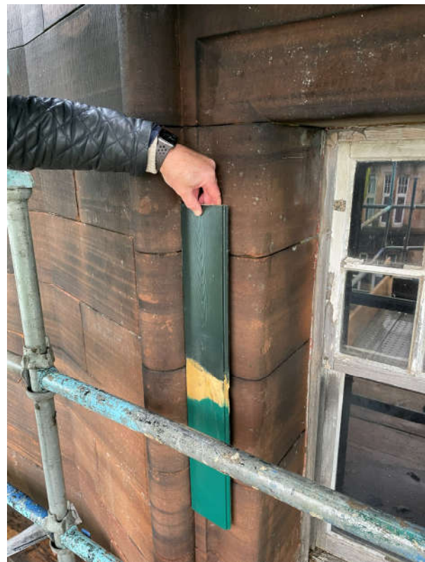
9005-B80G above, 6030-B90G below. The paint samples were reviewed against the stone to ensure they complemented its tone and achieved the appropriate heritage appearance. The upper sample, 9005-B80G, was considered the most suitable.
