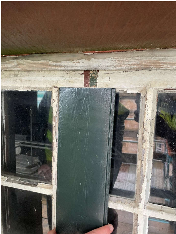
Sample of colour 9005-B80G to an alternative window test area again showing a close visual match
