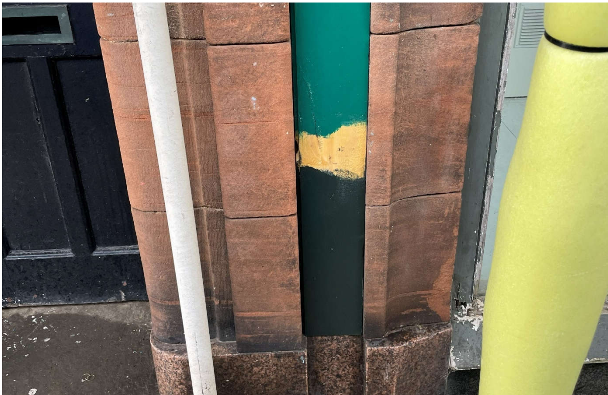
The samples—6030-B90G above and 9005-B80G below—were reviewed in a separate location to assess their suitability and determine which provides the best heritage appearance and contributes positively to the streetscape. The lower sample, 9005-B80G, was considered the better choice, offering a richer tone that will enhance the heritage character of the windows and make a positive contribution to the streetscape.
