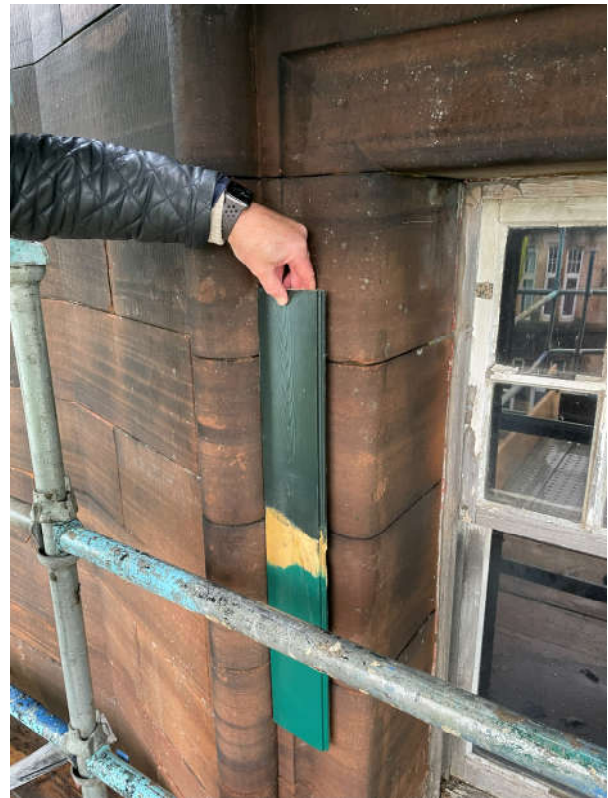
9005-B80G above, 6030-B90G below. The paint samples were reviewed against the stone to ensure they complemented its tone and achieved the appropriate heritage appearance. The upper sample, 9005-B80G, was considered the most suitable.
