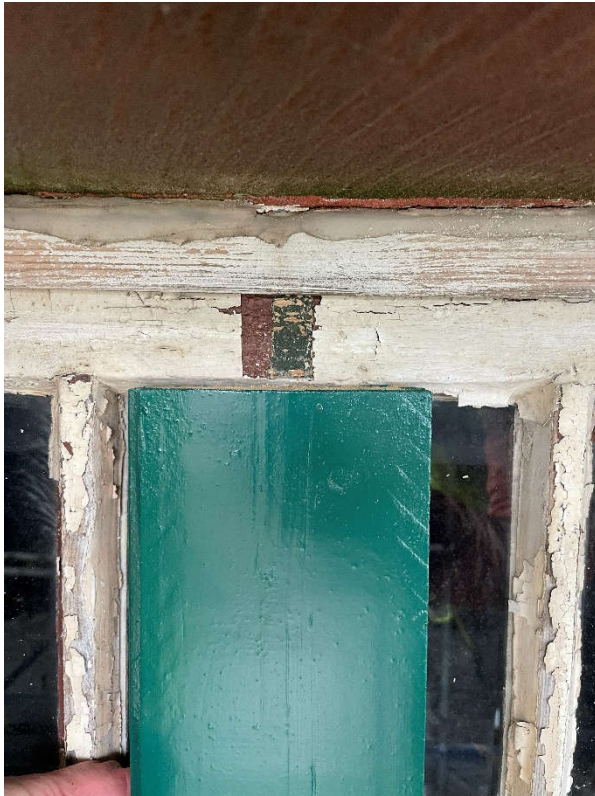
Sample of colour 6030-B90G. It was identified as not being a good match to the existing colour being more mid green.
