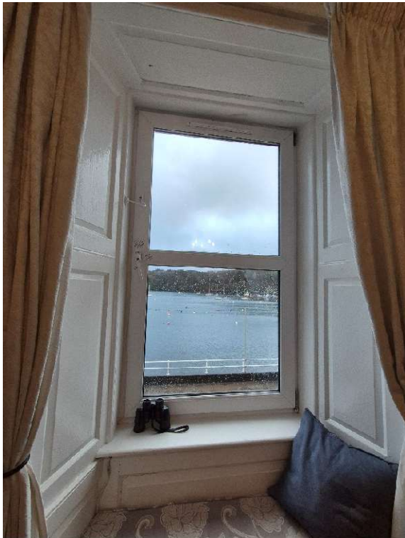
Fig 2 shows the window from the inside of the property.
