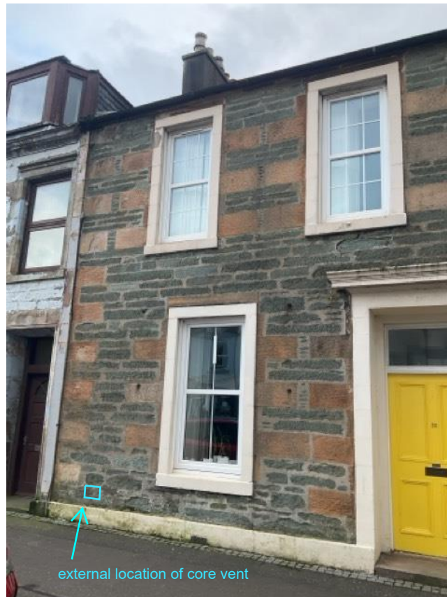
Living Room Combustion Appliance Core Vent Location
