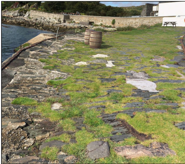
Figure 6: Ardbeg Distillery Sea Wall and Pier today, ca. 2018 (c) Google
