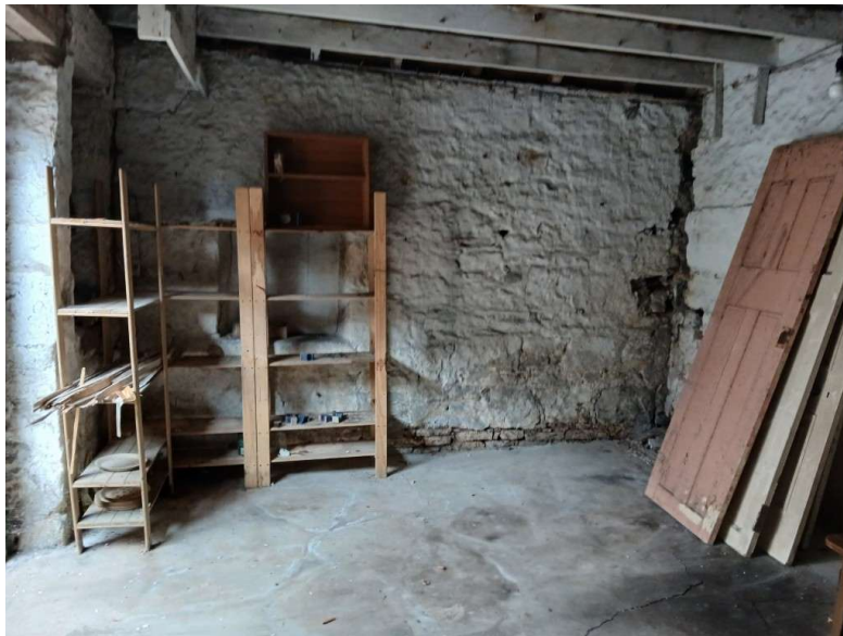
Photograph No.22 – Eastern gable wall. Concrete slab sloping towards northern side.
