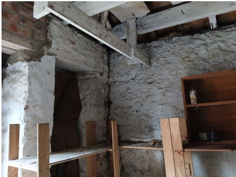
Photograph No.24 – Opening up at intersection of north and east walls.
