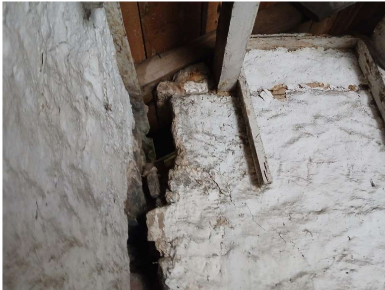
Photograph No.20 – Close up of head of wall as photo 19.
