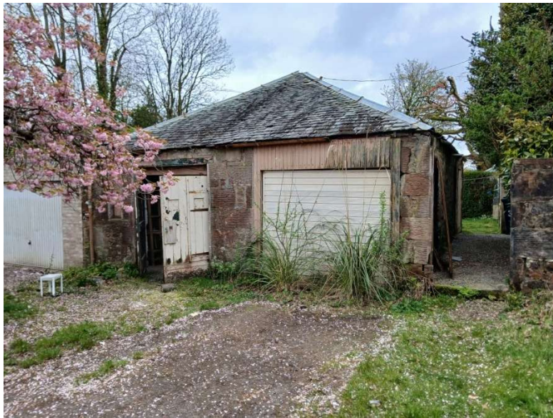
Photograph No.6 – North (road) elevation.
