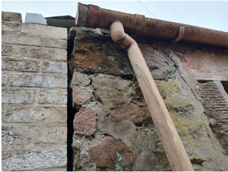
Photograph No.7 – Close up of head of north-eastern corner adjacent to neighbouring property.
