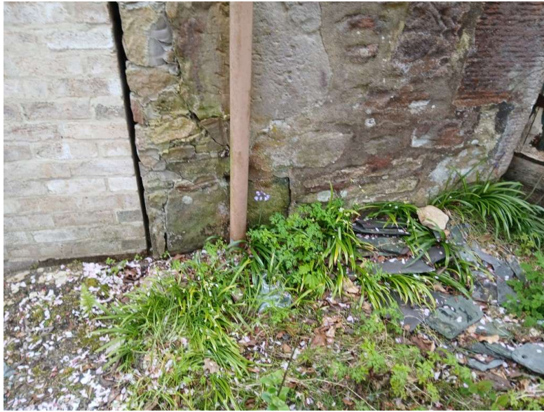
Photograph No.9 – Base of wall below photo 7 & 8.
