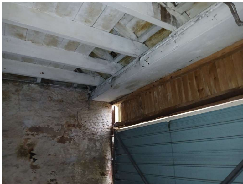
Photograph No.26 – Timbers to roof appear in reasonable condition. Safe lintol not visible condition unknown.
