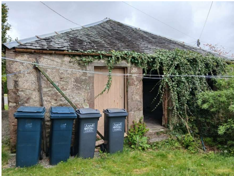
Photograph No.2 – South (rear) elevation.
