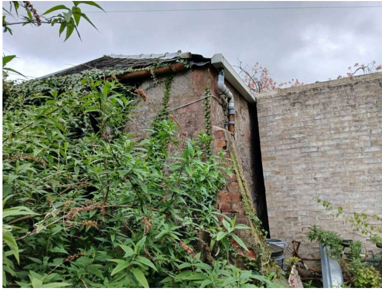
Photograph No.1 – Partial East Elevation not obscured by neighbouring garage.
